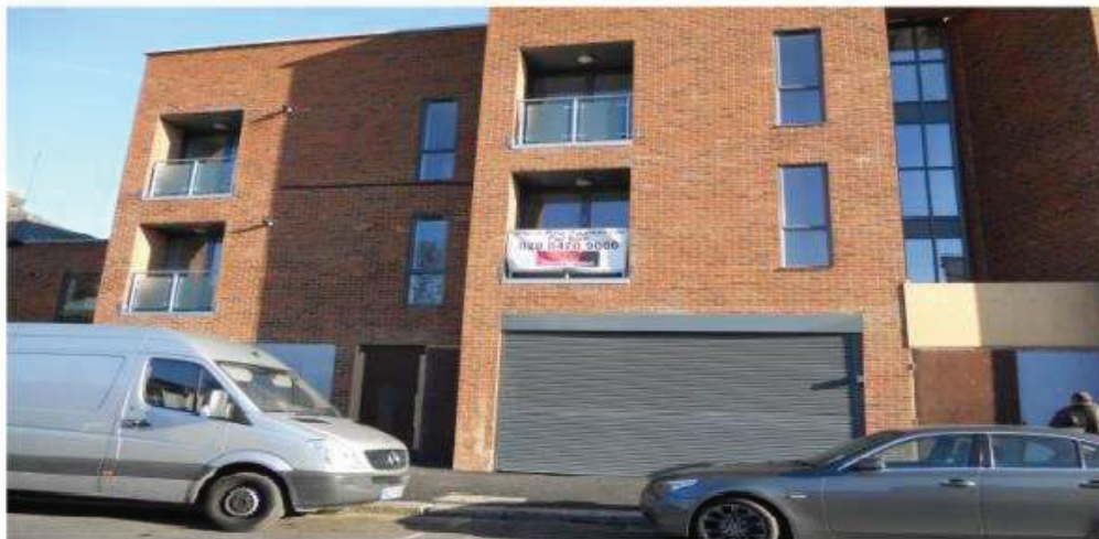
HOTEL RAILING WINDOW SOLUTION, LONDON, UK
