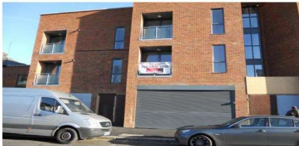
HOTEL RAILING WINDOW SOLUTION, LONDON, UK
