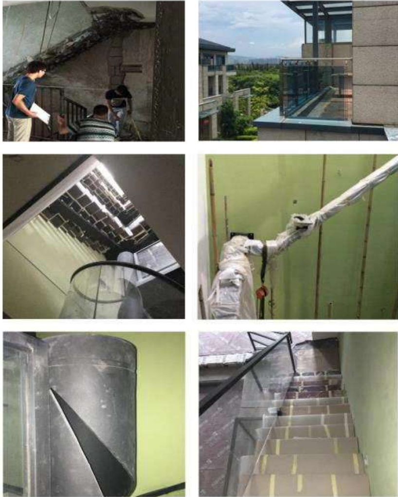
VILLA MARINE GRADE SS RAILING STAIR SOLUTION, SHENZHEN
