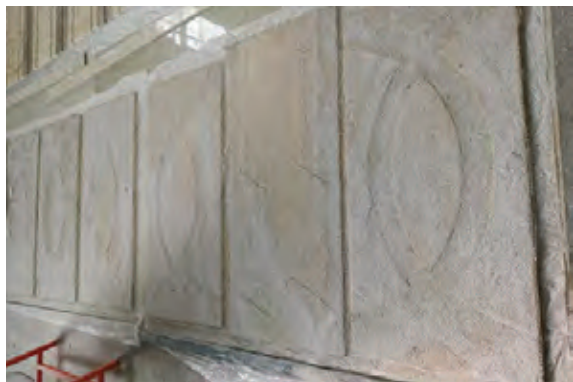
9. Leveling the pattern by net and sand
