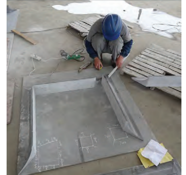
4. Process of jointing
